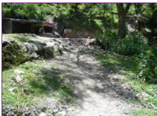
Starting point of Approach Road to Dam site
