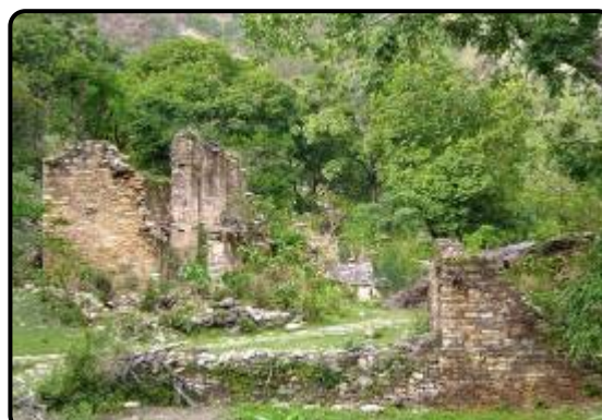
Remains of abandoned double storied guest house (Heritage building) on Haat- Siyasain ancient route
