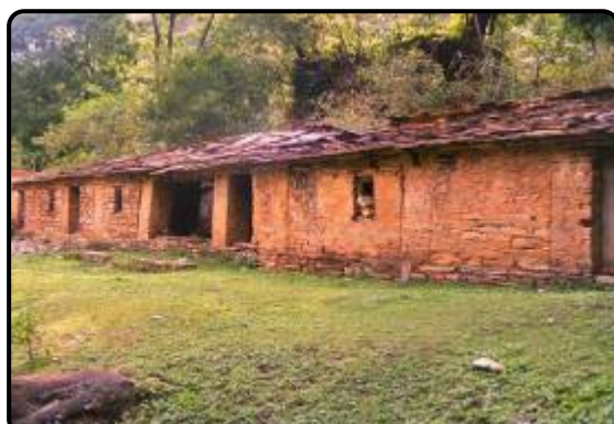
Abandoned shops (Heritage buildings) Siyasain ancient Route to Badrinath
