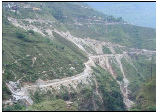
Approach Road to Maina Adit
