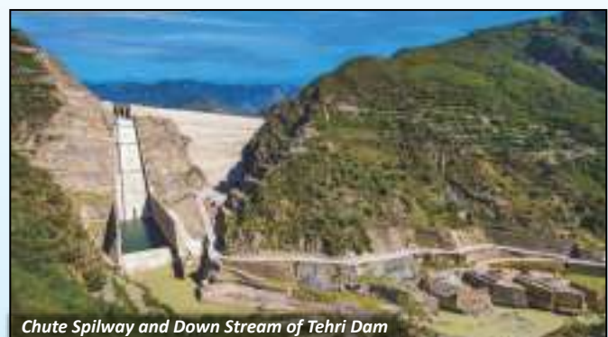
Chute Spillway and Down Stream of Tehri Dam
