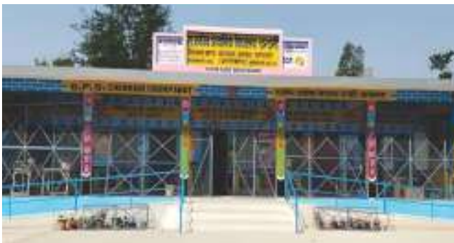
Reconstructed Govt. Primary School, Chandini (Dist. Champawat), Uttarakhand.
