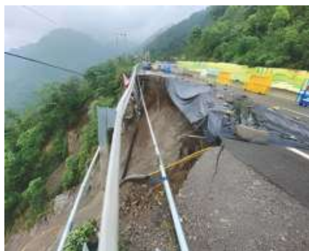
Fig.-10: Loss of valley side portion of the pavement
