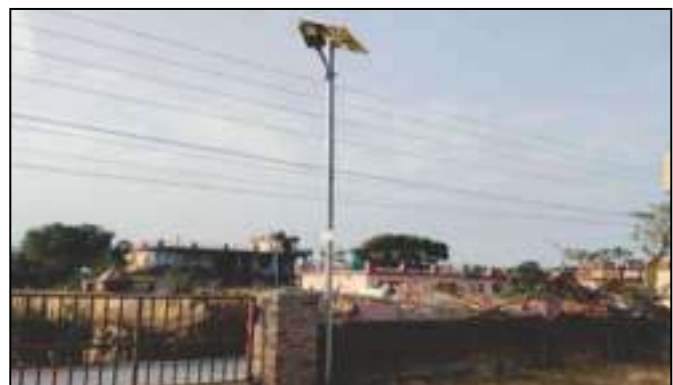
Installation of Solar Street Light at Rishikesh
