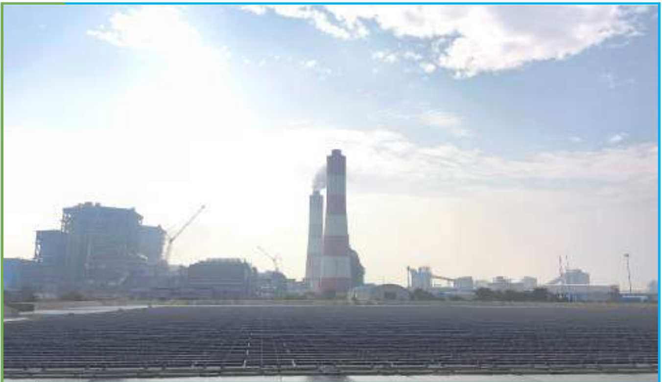
1320 MW Khurja Super Thermal Power Plant
