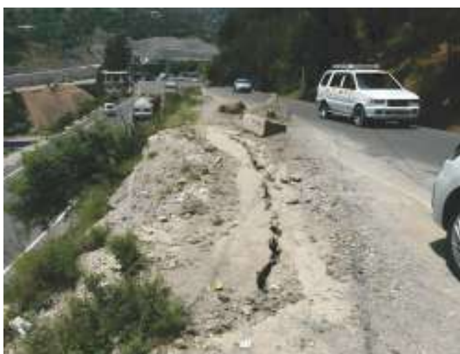
Fig.-9: Valley side movement of detached mass
