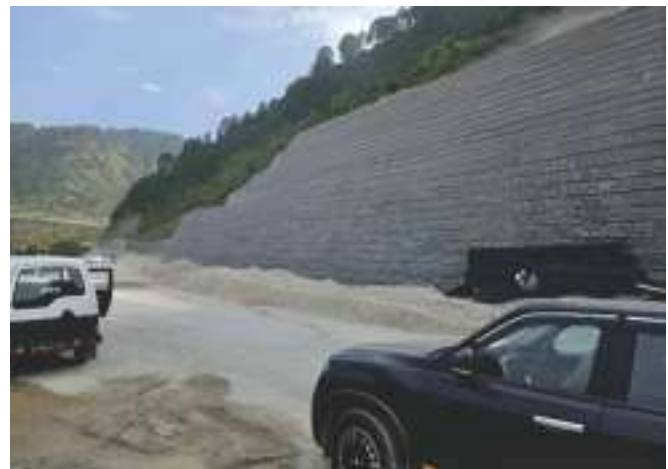
Fig.-6: RS wall with welded mesh facia under construction at Chinnyalisour, Uttarakhand along NH-34
