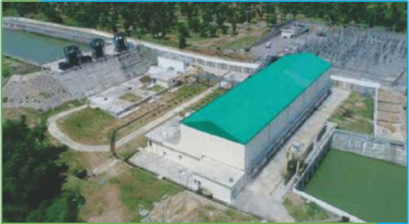
Aerial view of 24 MW Dhukwan SHEP
